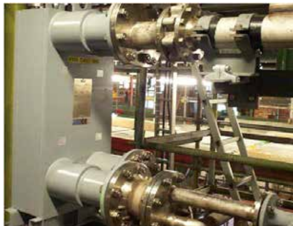
SIGMA WIG ST30 for steam condensation
