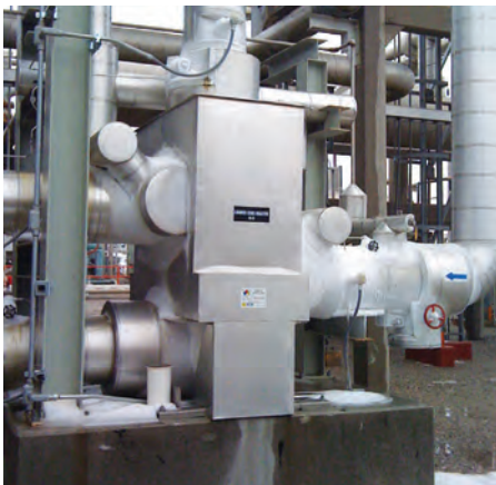
Reducing maintenance as a demethanizer low side heater replacing brazed units.
